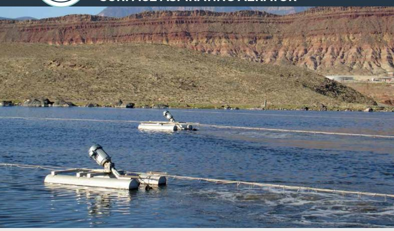
Powerful and reliable, self-aspirating surface Tornado aerators are used to upgrade lagoon systems and expand the treatment capacity of mechanical wastewater treatment plants.
